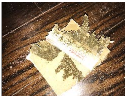
Photo 12 – Mould growth identified on wall finishes on the east wall inside Unit 200 and on the south wall outside the entrance of Unit 200.
