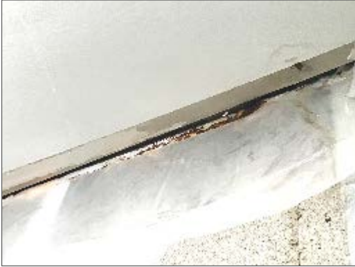
Photo 17 – Rusty metal framing and stained drywall ceiling identified in the 2 nd Floor Hallway.
