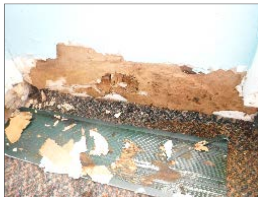
Photo 16 – Mould growth identified on the wall finishes along the south wall of Unit 202.
