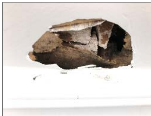
Photo 14 – Mould growth identified along the west wall of Unit 203.
