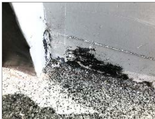
Photo 10 - Mould growth on wall finishes along the east wall of the Lobby.
