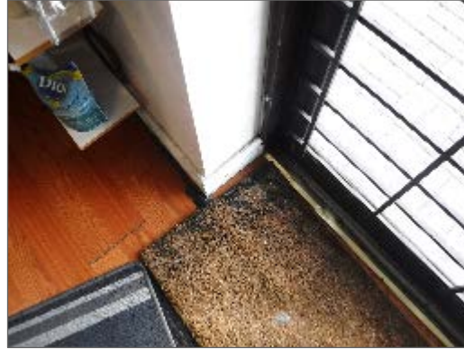
Photo 4 – Wet wall finishes identified in Unit 102.
