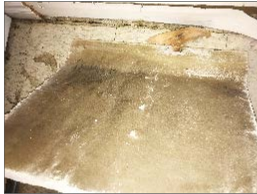
Photo 8 – Mould growth on wall finishes along the north wall of Unit 104.
