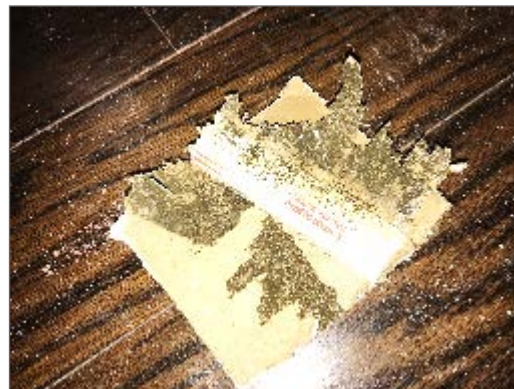
Photo 12 – Mould growth identified on wall finishes on the east wall inside Unit 200 and on the south wall outside the entrance of Unit 200.
