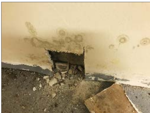
Photo 23 – Mould growth on a drywall wall in the northwest room.
