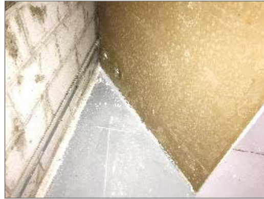
Photo 26 - Mould growth on the backside of the drywall along the west wall of the east room.
