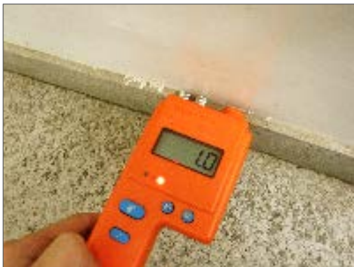
Photo 1 – Wet wall finishes identified in Washroom 1 of Unit 101.
