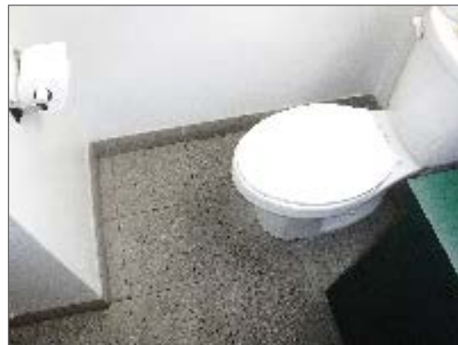
Photo 2 – Wet wall finishes identified in Washroom 1 of Unit 101.
