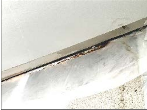
Photo 17 – Rusted metal framing and stained drywall ceiling identified in the 2 nd Floor Hallway.
