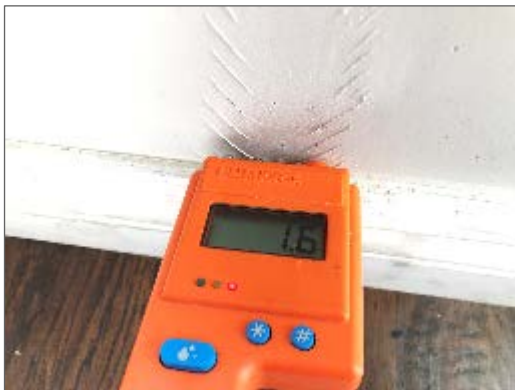
Photo 13 – Wet wall finishes along the west wall of Unit 201.
