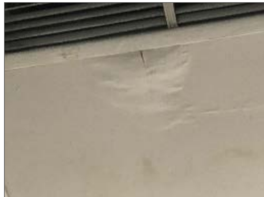
Photo 22 - Water damaged drywall ceiling in the 2 nd Floor Hallway outside of Unit 202.
