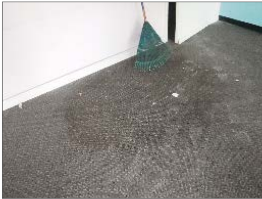
Photo 15 – Water stained carpet on the north side of Unit 202.
