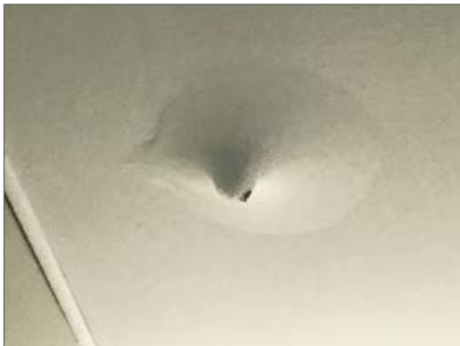
Photo 21 – Water damaged drywall ceiling in the 2 nd Floor Hallway outside of Unit 202.
