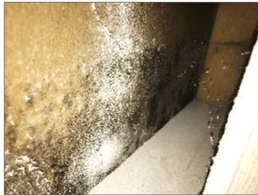
Photo 6 – Mould growth on the wall finishes along the north wall of Unit 103.
