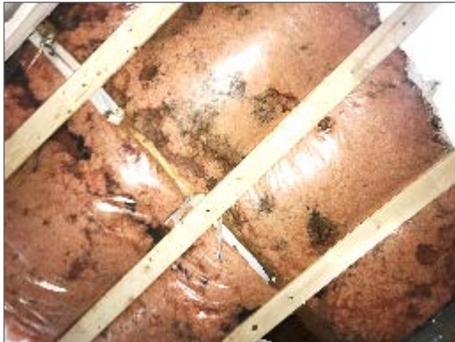
Photo 19 – Exposed ceiling exposing stained fiberglass insulation and water damaged drywall.
