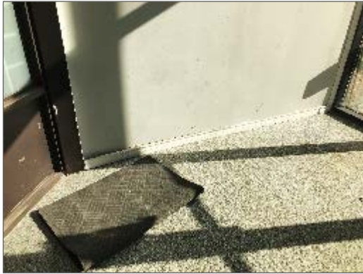
Photo 9 – View of the east wall in the Lobby where mould growth is present.
