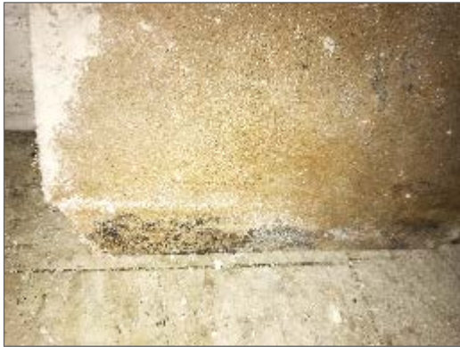
Photo 7 – Mould growth on wall finishes along the east wall of Unit 104.
