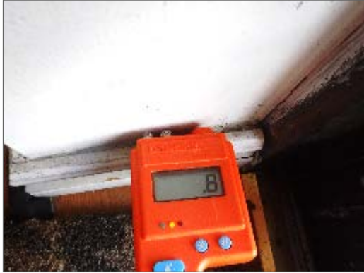
Photo 3 – Wet wall finishes identified in Unit 102.
