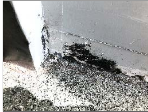
Photo 10 - Mould growth on wall finishes along the east wall of the Lobby.
