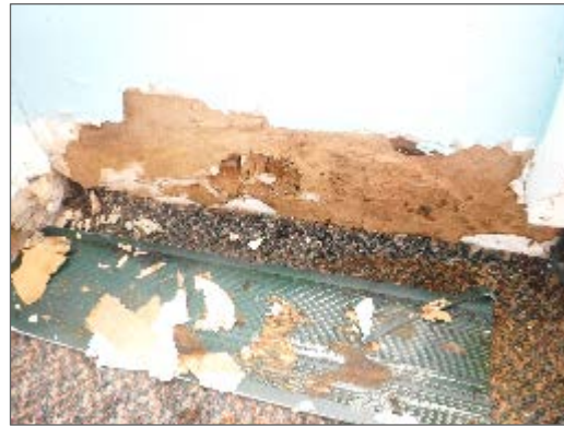
Photo 16 – Mould growth identified on the wall finishes along the south wall of Unit 202.
