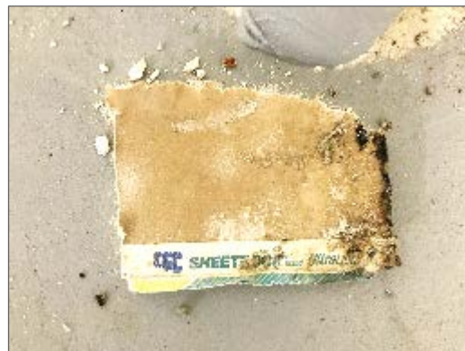
Photo 24 - Mould growth on a drywall wall in the northwest room.
