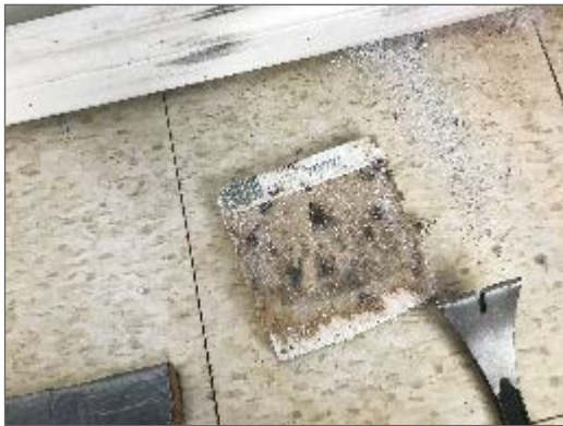
Photo 5 – Mould growth on wall finishes along the south wall of Unit 104.
