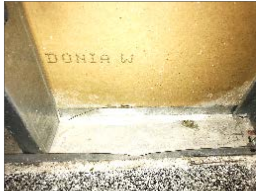
Photo 20 – Mould growth on drywall on the backside of the Women's Washroom.
