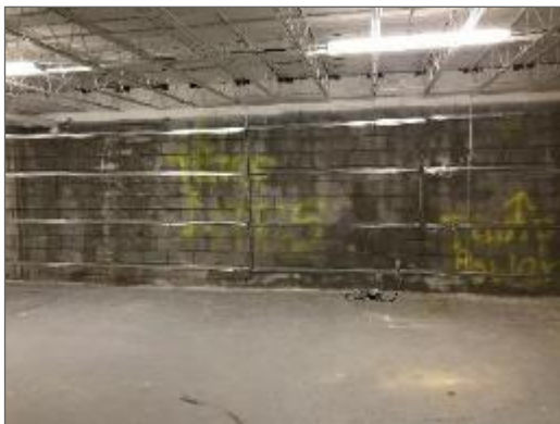
Photo 27 – Staining and efflorescence on exposed concrete block wall.
