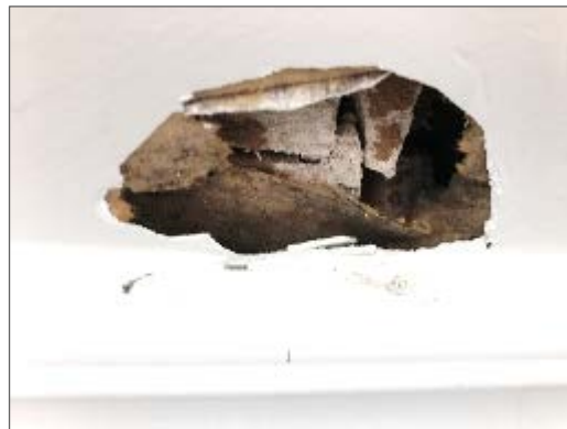
Photo 14 – Mould growth identified along the west wall of Unit 203.
