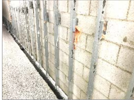
Photo 18 – Sections of the wall finishes have been removed to full height in the 2 nd Floor Hallway.
