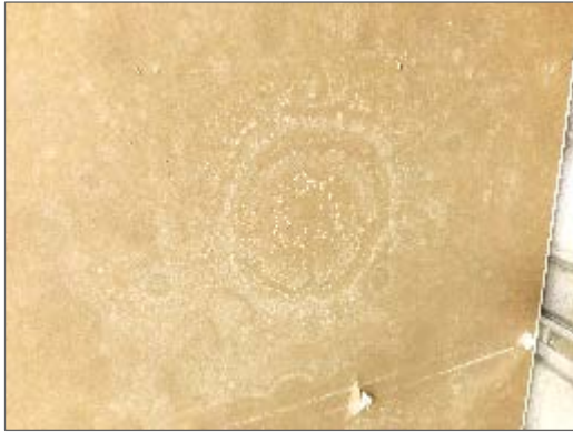
Photo 25 – Mould growth on the backside of the drywall along the west wall of the east room.
